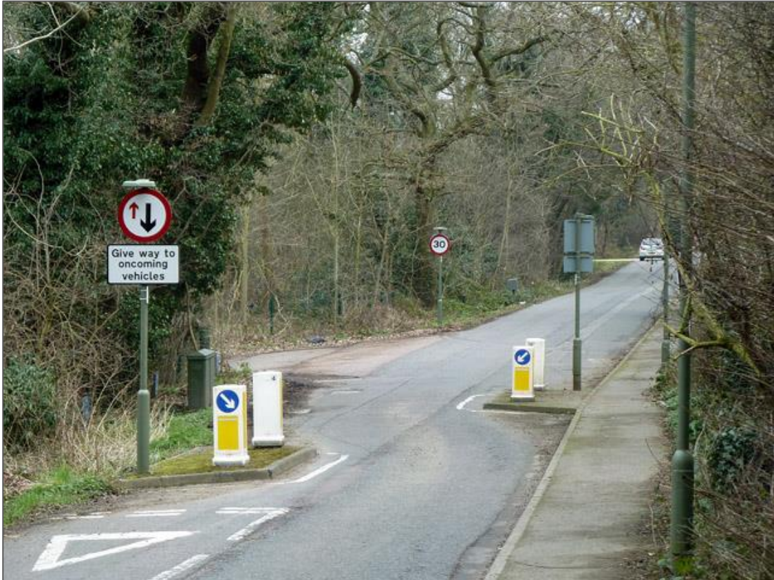
Figure 3: Indicative example of a double build-out chicane
